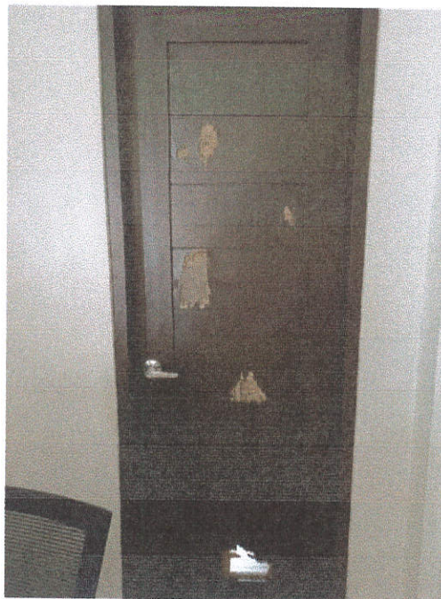
Damaged wooden door at quarter's area toilet for replacement
