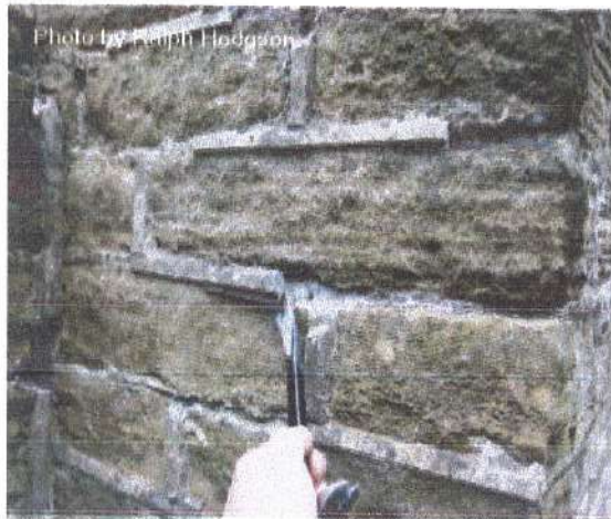
Repointing techniques of stone masonry
