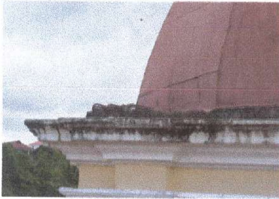
Black deposits at the ledges of the bell tower & cornice
