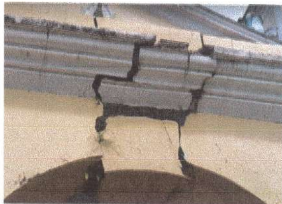
Damaged masonry units for retrofitting
