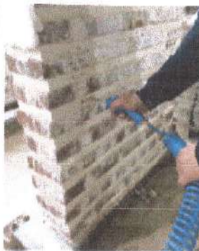
Lime water consolidation technique procedure
