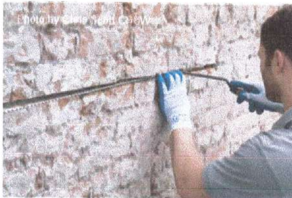
Stainless steel helical rod installation to reinforce masonry walls
